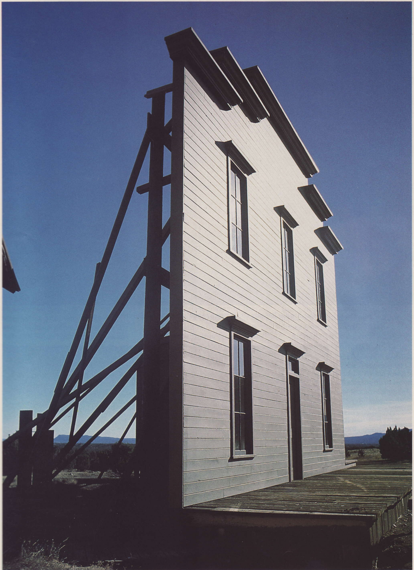
Buildings at the Eaves Movie Ranch look authentic, but a step to the side reveals that some are actually false-front structures.
